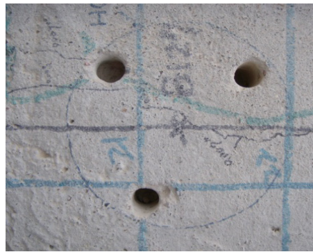
Figure 3.17. Photograph of three holes drilled to collect concrete powder within a 4-in. diameter.
