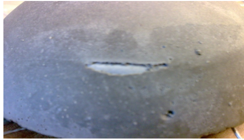
Figure 4.27. Observed spalling of cement paste cover (Sensor J005).
