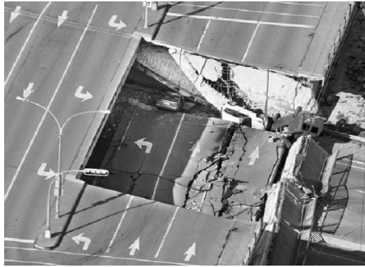
Figure 1.1. Collapse of a highway overpass near Montreal, Canada (From New Civil Engineer Magazine 2006)
