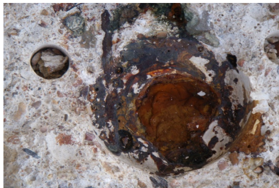
Figure 3.20. Photograph of the corrosion directly below Sensor B135.
