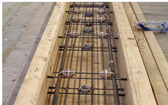
Figure 3.5. Photograph of the layout of the sensors and steel reinforcement (Puryear 2007).
